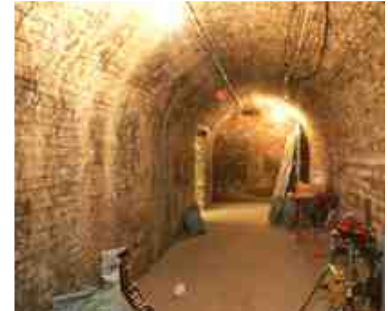
Newtonite lath removed to original substrate.
