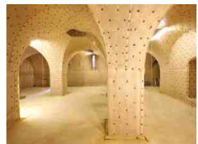
Membrane fully installed, in preparation for a direct render finish.
