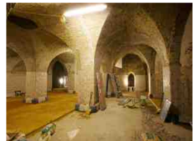
Membrane and drainage system installation in progress.
