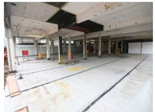
System installed throughout entire basement floor.
