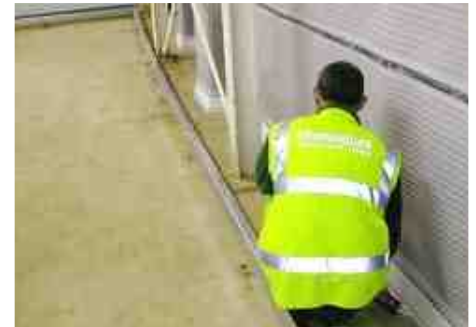
Newton Baseboard applied to RC wall.
