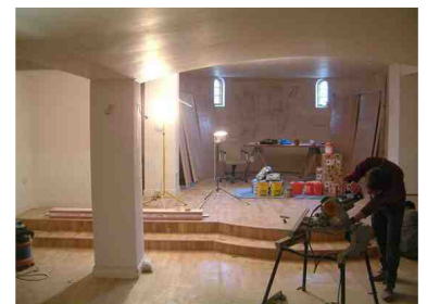
Moisture sensitive flooring installed over Slimline Floor membrane.
