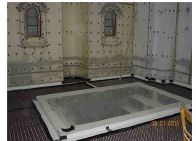
All Newton membrane products were installed within this complex waterproofing project.
