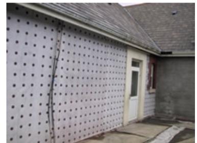
Applying Newlath 2000 damp proofing membrane to walls.
