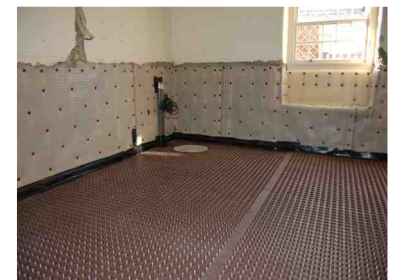
Newton 520 applied to floor area.
