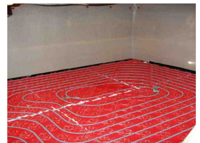
Underfloor heating installed prior to screed finish.
