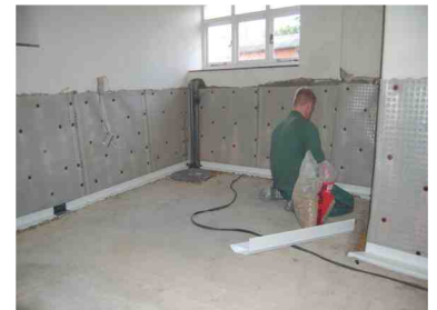
Wall membrane and basedrain installation.
