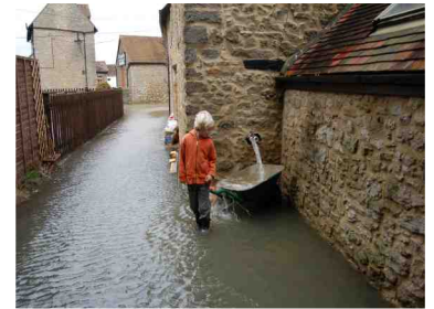
Newton system being tested in flooding conditions.
